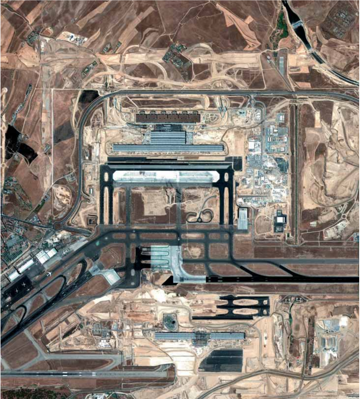
Aerial view of the site during construction of the new terminal building and satellite
