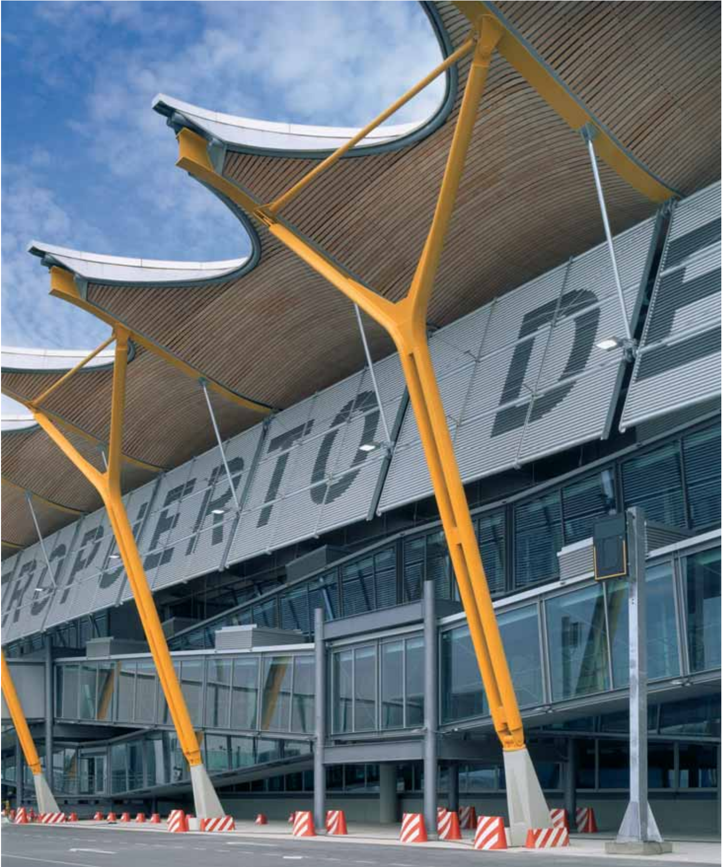
New Area Terminal (NAT) Barajas Madrid, Spain 1997 - 2006
