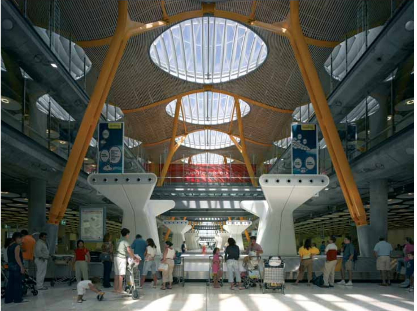
The baggage reclaim hall showing the air-conditioning units integrated into the reclaim units
