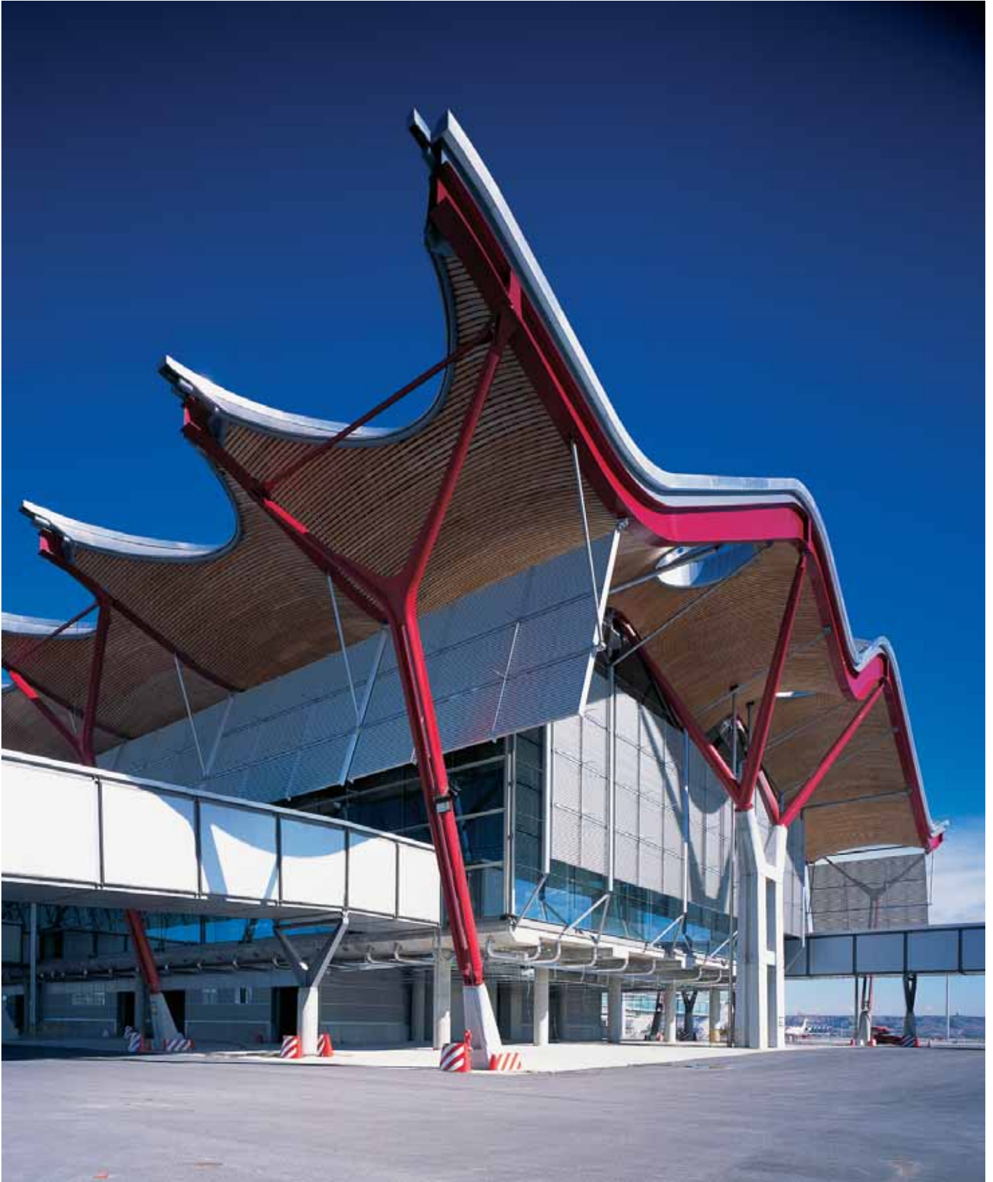
New Area Terminal (NAT) Barajas Madrid, Spain 1997 - 2006
