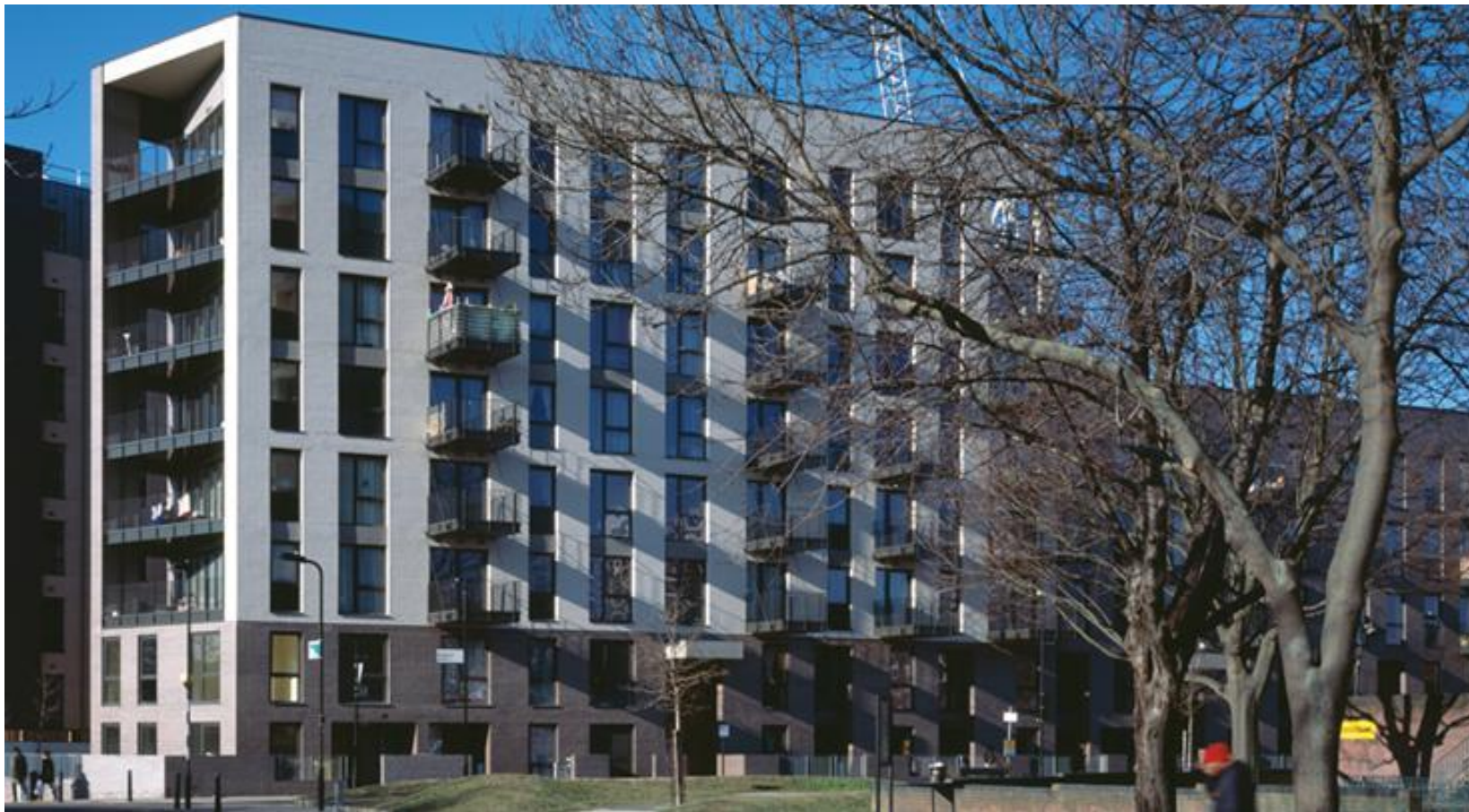
Bridport House, east London, by Karakusevic Carson Architects
