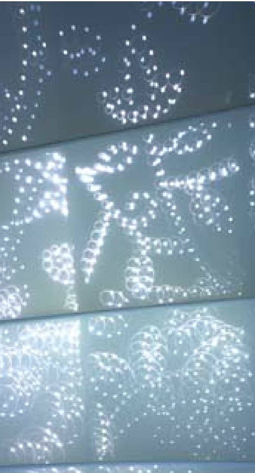
4700 holes make a lacelike drawing on the steel leaf
