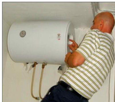
18 · Procedures for Commercial Building Energy Audits
