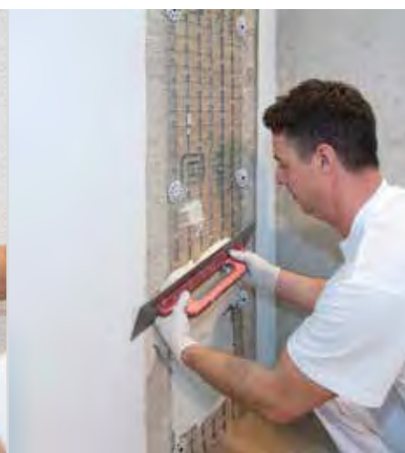
Elaborare (RÖFIX Stucanet) ponte fessure
